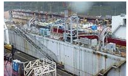
Worker on gangway between edge of floating dry dock and vessel
